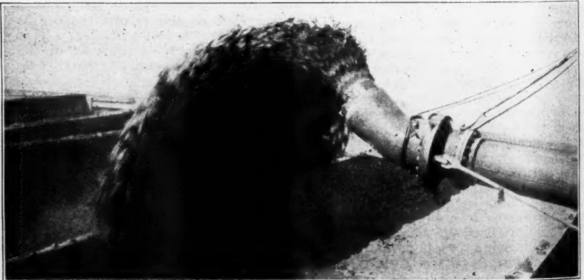
Pumping Oyster Shells Into Barge
